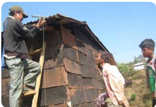
Photo No 3: Tying Roof of a House to reduce the impact of Cyclone
